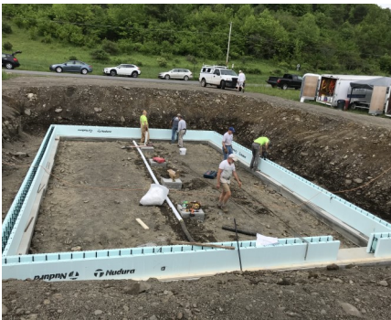
Installing the foundation using ICF forms at lot four on McFar.and Rd. .
