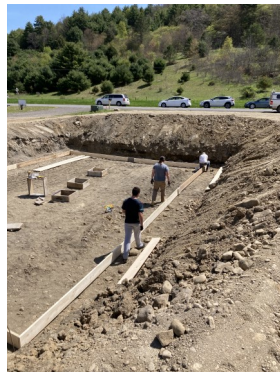
Installing the foundation using ICF forms at lot four on McFar.and Rd. .
